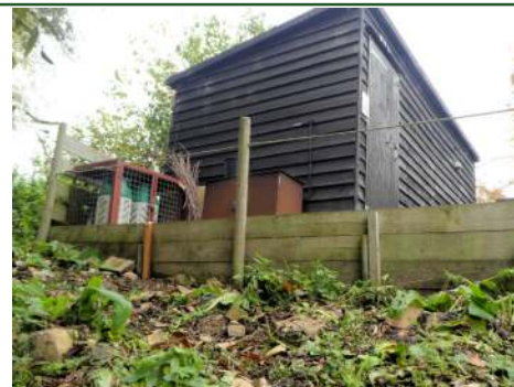
The new retaining wall
