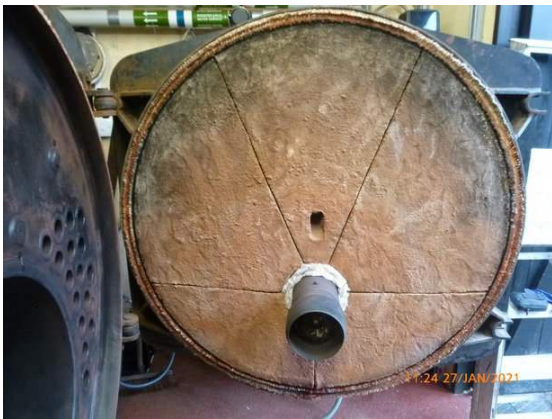
Inside of boiler door
