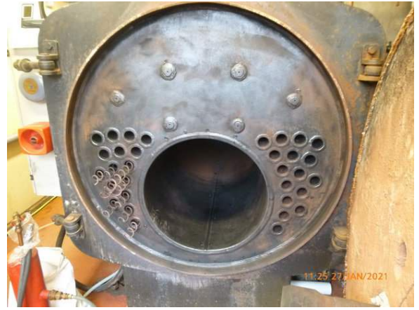
Boiler tubes ready for inspection
