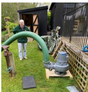
We took delivery and installed a new river pump to drive the waterwheel
