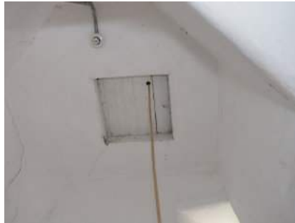
View up to trap door to access bell
