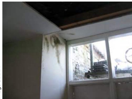
Typical damp patches around toilet window plus deteriorated paint to obscure the window
