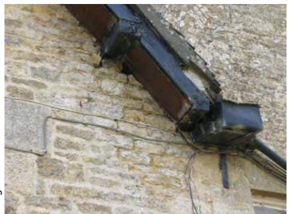
Rotten timber in edge of front roof and cracks in rubble wall
