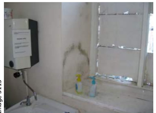
Typical damp patches around toilet window plus deteriorated paint to obscure the window
