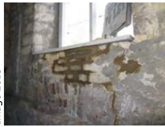
Stonework beneath staircase window sill - replaced in 2008
