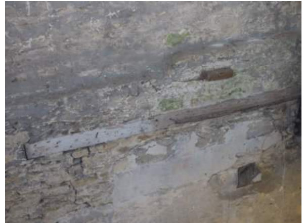
All wall plate timbers repaired and rafters partnered with new timber where needed
