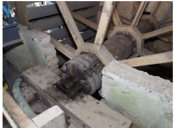
Waterwheel gudgeon bearings re-wedged and steel banded
