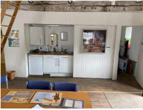
New kitchenette/ bookshelves installed under steel beam
