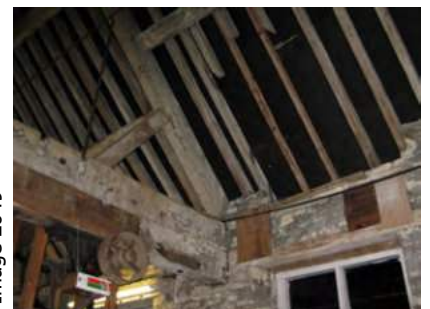
Above window showing roof construction where once a dormer light existed - this is the case for each alternate window bay
