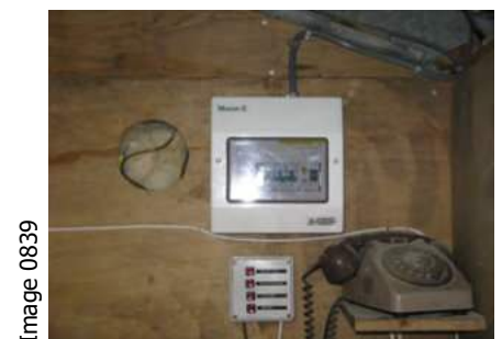
Board C - boiler house and disabled toilet
