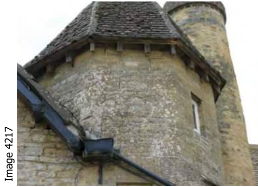
Crack in wall of turret
