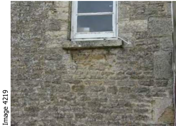
Cracks in rubble wall below front window of Education Room
