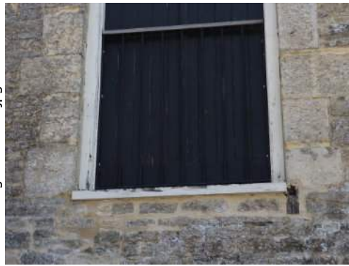
View of yard wall - loading bay door repaired timber and stonework
