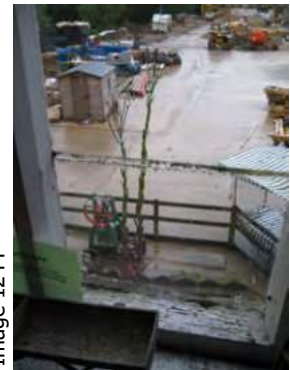
Weed growing on outside of rotten window sill
