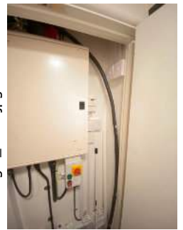
Distribution board in Tea Room - feeding river pump and two storage sheds
