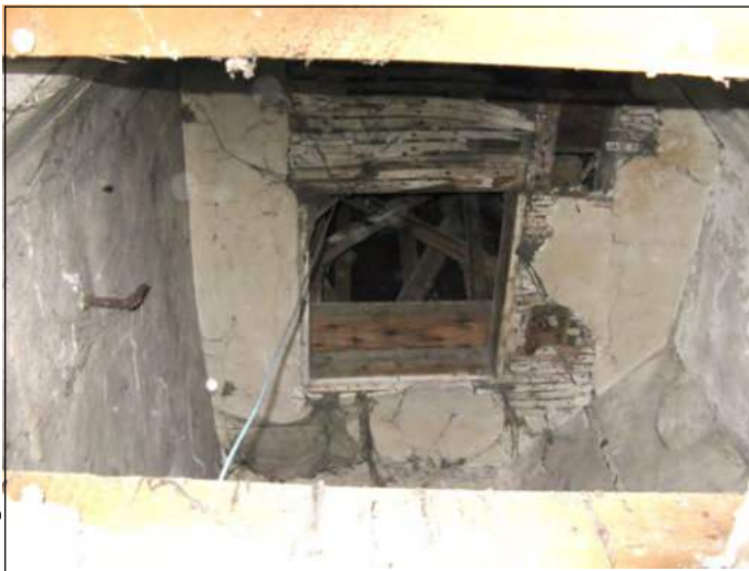
Another view up into bell tower through hatch
