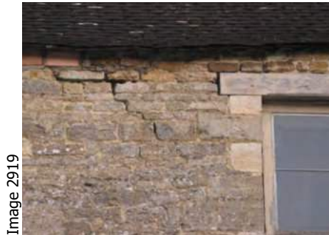
Typical state of rubble walls showing another strengthening plate and cracks
