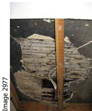
State of toilet ceiling before re-plastering in June 2009
