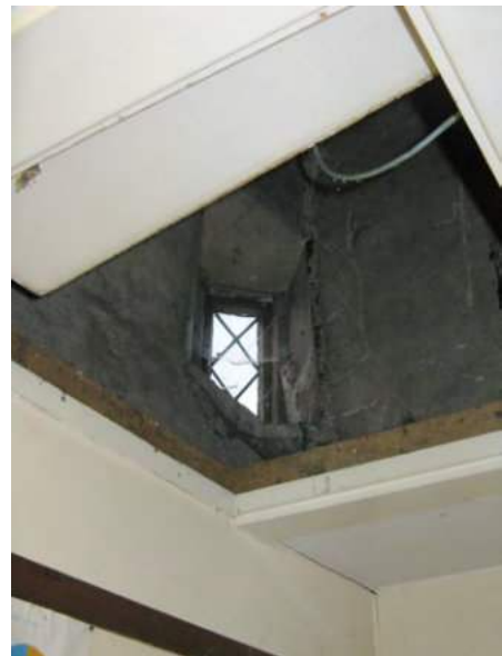
View through hatch of turret window
