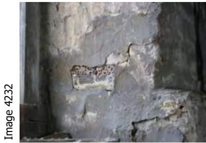
Old timber embedded in stonework
