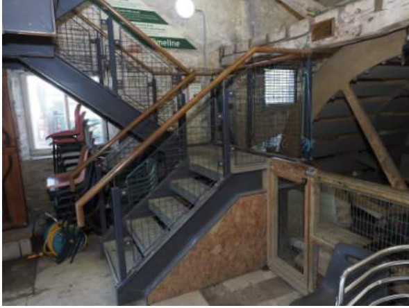
Old wooden staircase replaced with steel
