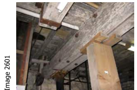
Prop beam in workshop
