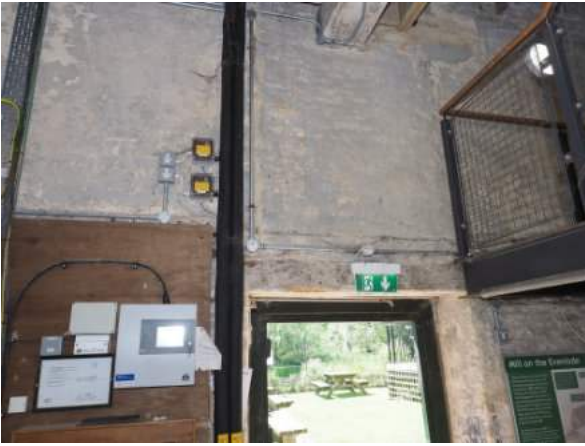
Stonework crack above door repaired
