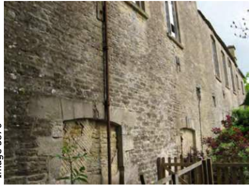
Further images showing lack of guttering, broken stone window lintels and cracks in rubble wall
