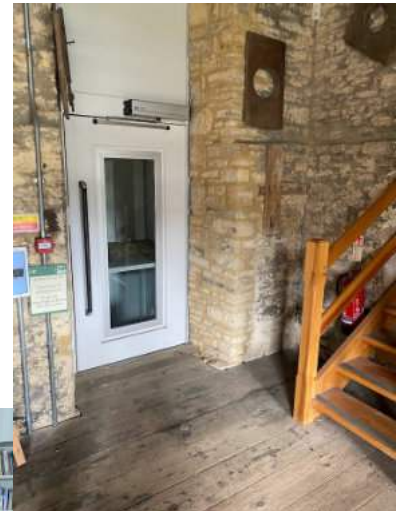
Lift landing on second floor - was a window opening
