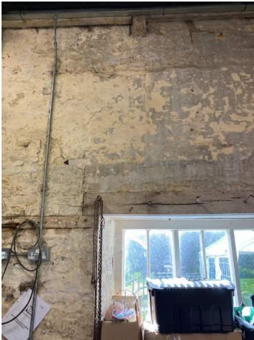
Stonework crack above window repaired
