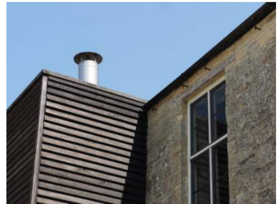
Boiler flue via lift shaft housing
