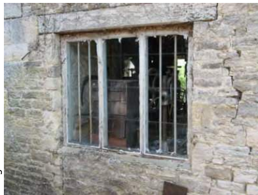
Workshop window to left of rear forge door with associated cracks and distressed timber lintel
