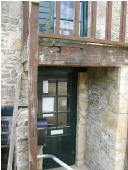
Split wooden support upright of staircase
