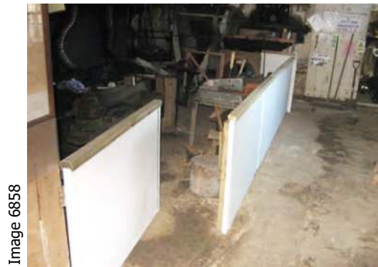
Spark resistant safety barriers across forge area erected February 2008
