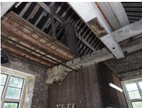
Old roof slates replaced with tiles in this quarter of roof
