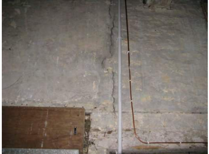
Vertical crack in wall above end door rising through floor above
