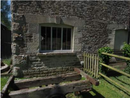
Repaired window of waterwheel room
