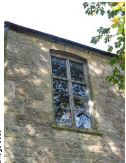
Series of images showing lack of guttering, broken stone window lintels and cracks in rubble wall
