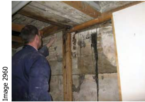
State of wood rot adjacent old sawmill before re-plastering in June 2009
