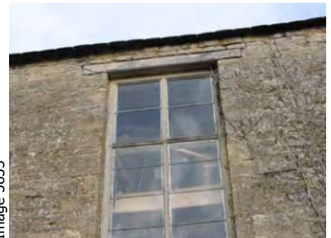
Typical state of windows - timber unpainted - large gaps around edges - poor glazing
