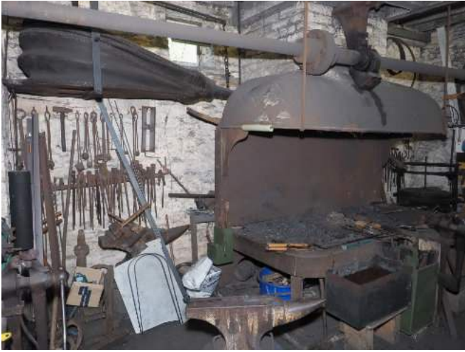
Flexible metal extract ducts removed together with electric extract fan housed in hood
