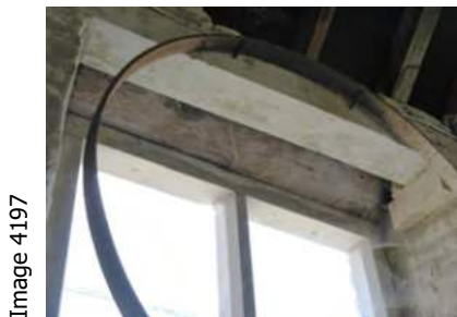
Another window lintel with signs of wood rot
