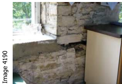
Window sill replaced with cement in the past and state of stonework surround - in refreshment area
