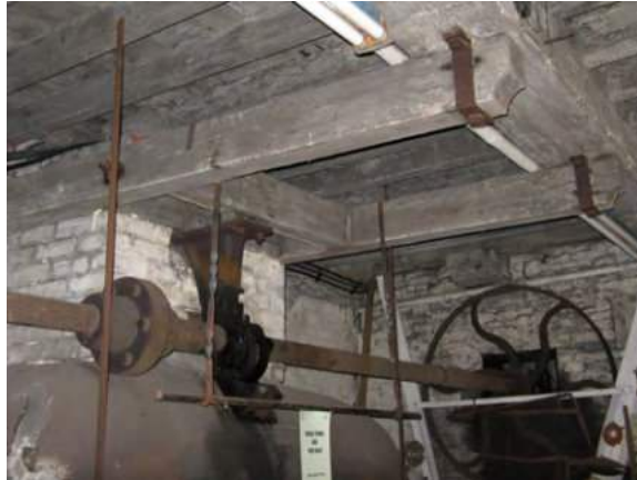
Views showing ceiling beams in forge/workshop
