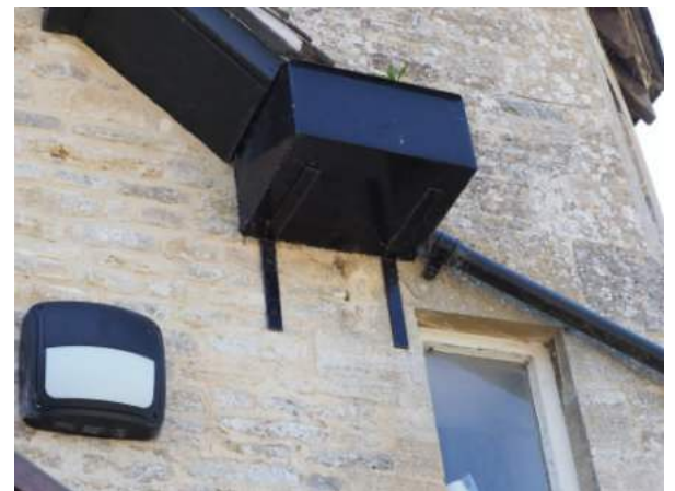
Replaced rainwater tundish
