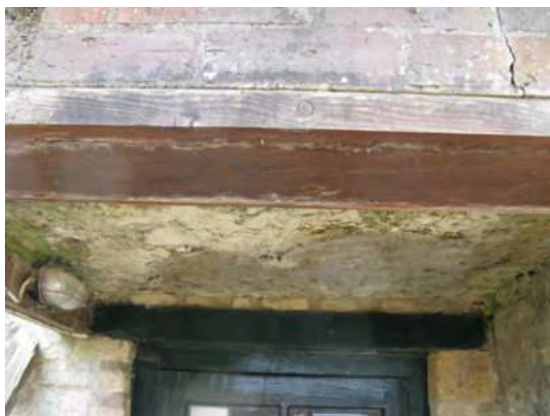
Crumbling slab of staircase landing
