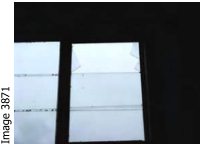
Broken glass pane - typical
