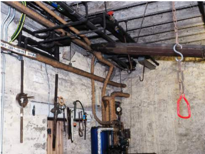
Steam pipework re-routed and lagged with fibre.
