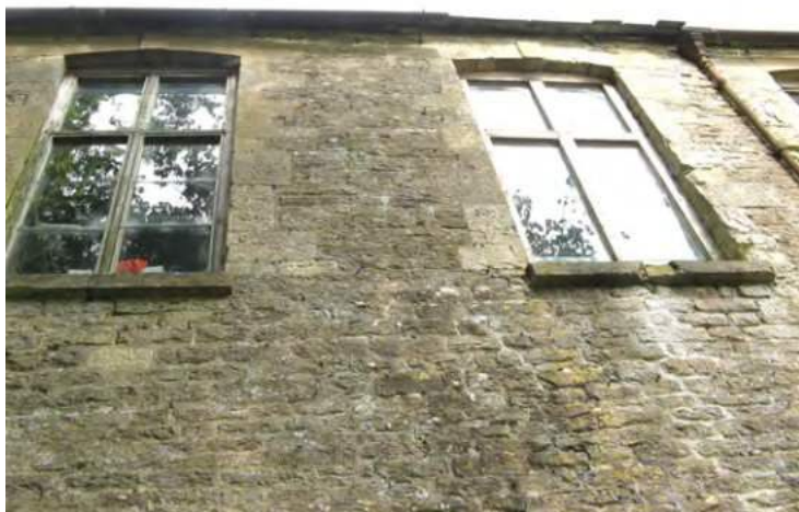
Series of images showing lack of guttering, broken stone window lintels and cracks in rubble wall
