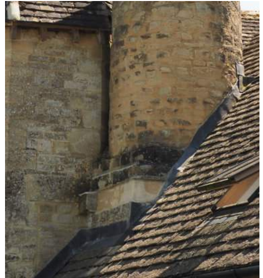
Repaired stonework at chimney base
