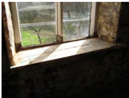
State of Engine Room window showing ill fitting metal frame and repaired window sill
