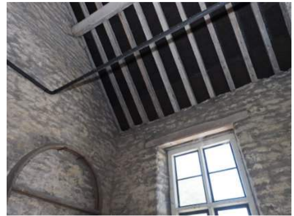
All wall plate timbers repaired and rafters partnered with new timber where needed
