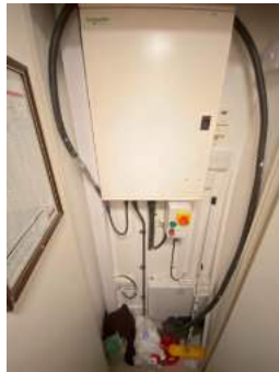
Distribution board in Tea Room - feeding river pump and two storage sheds
