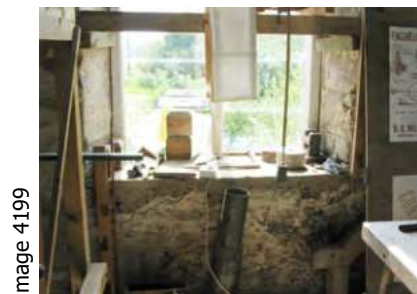
Window sill behind historic clock display repaired with cement
