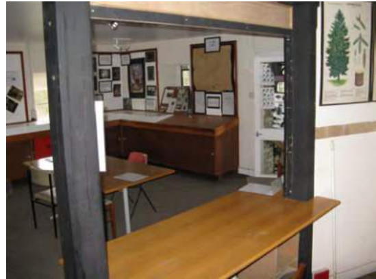
View into education room from 'corridor' - the two vertical black columns support the structurally weakened main beam that carries the turret
