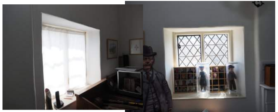
Remaining leaded window retained and refurbished.
