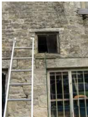
Small vent above rear forge door and associated cracks and distressed timber lintel
