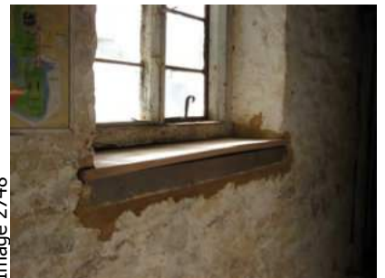
State of Engine Room window showing ill fitting metal frame and repaired window sill
