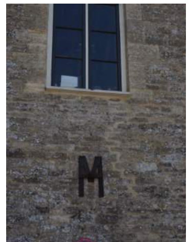
Showing repaired crack in stonework
