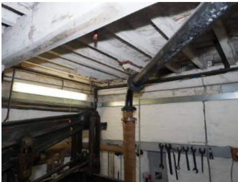
Steam pipe lagging replaced with fibre and metal cladding dispensed with.
