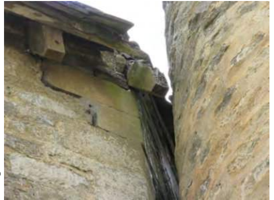
Damage to turret roof against chimney
