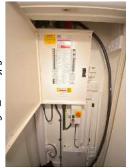
Distribution board in Tea Room - feeding river pump and two storage sheds
