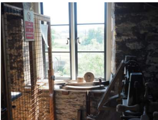
Stonework below window sills repaired throughout where necessary
