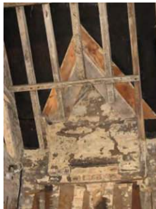
Roof beam arrangement around forge chimney
