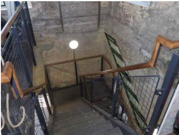
Old wooden staircase replaced with steel
