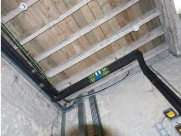
New cold water pipes lagged and heat traced
