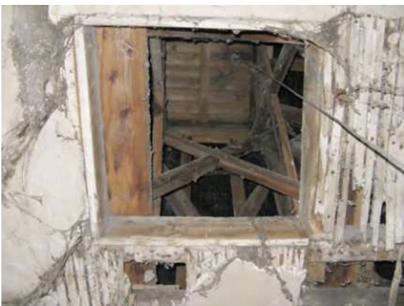
Framing of bell tower viewed through hatch
