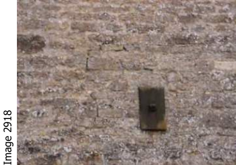
Typical state of rubble walls showing another strengthening plate and cracks
