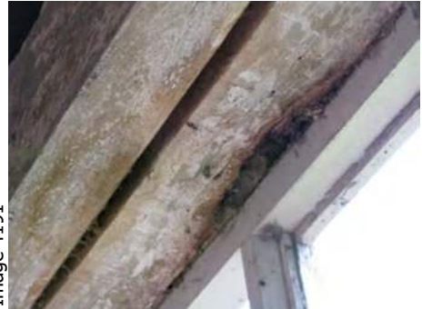
Gaps and rot around timber window frames
