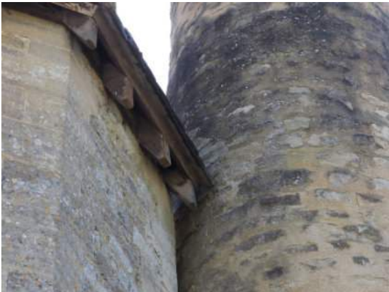
Repaired turret roof against chimney
