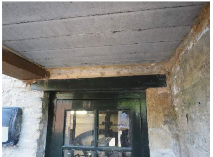
Repaired outside stairs landing
