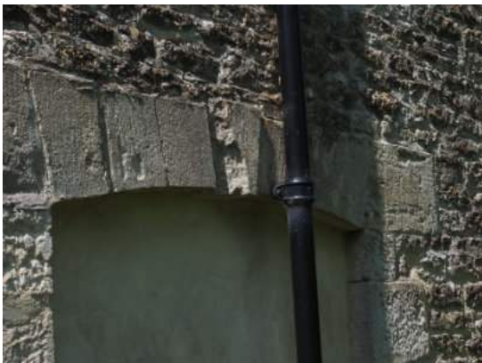
Repaired window of waterwheel showing stonework damage on keystone
