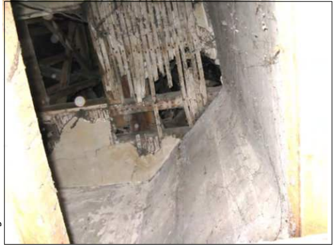
Inner ceiling laths of bell tower viewed through turret hatch
