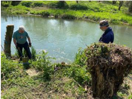
Keith Johnson and Alan Dear work to locate new paving slabs
