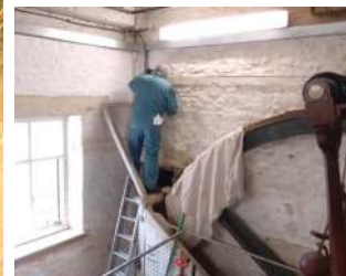
Engine room wall painting was completed
