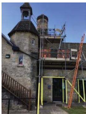
Chimney repairs completed
