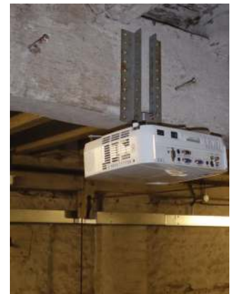
Projector suspended from timber beam
