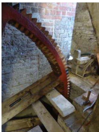
Section of refurbished pit gear
