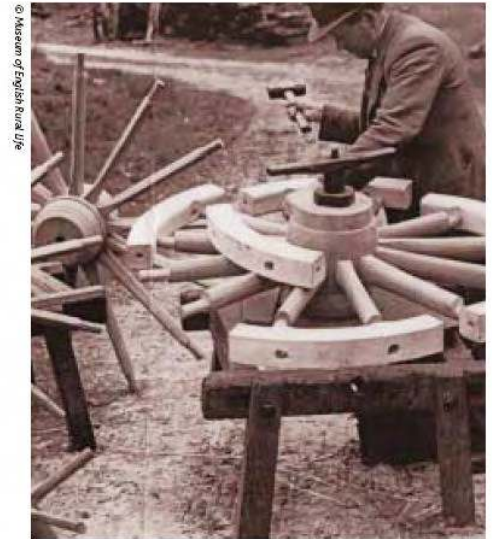
Hammering ash felloes onto spokes (1941)
